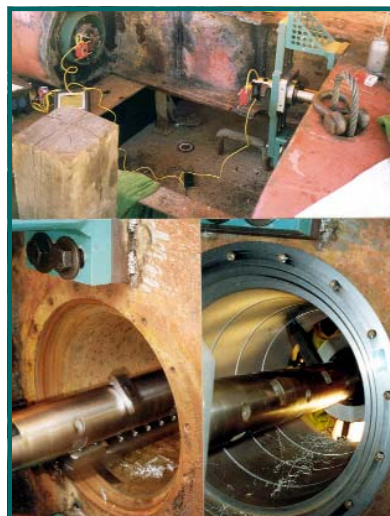
Ruderblatt, Kone bohren Boring rudder blade cones
